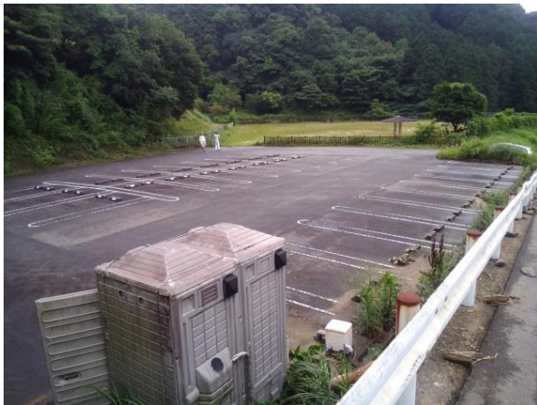
(仮置場開設前)
